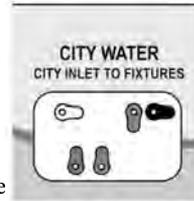
**NOTE:** To disconnect: Turn off water at the pressurized source first, disconnect hose from the water source, (to release pressure off the system) then disconnect the hose at the City Water Connection on Utility Center last.
